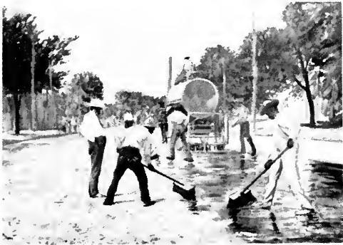
To combat the dust problem of the speeding auto on dry stone roads, the first Commission experimented with numerous oiling devices. This scene shows early application of coal tar and crude oil.
